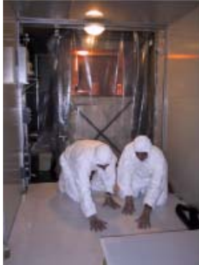
Figure 5: At work to improve the experimental site (walls, floor, etc.). On the bottom: the passive shield opened.
