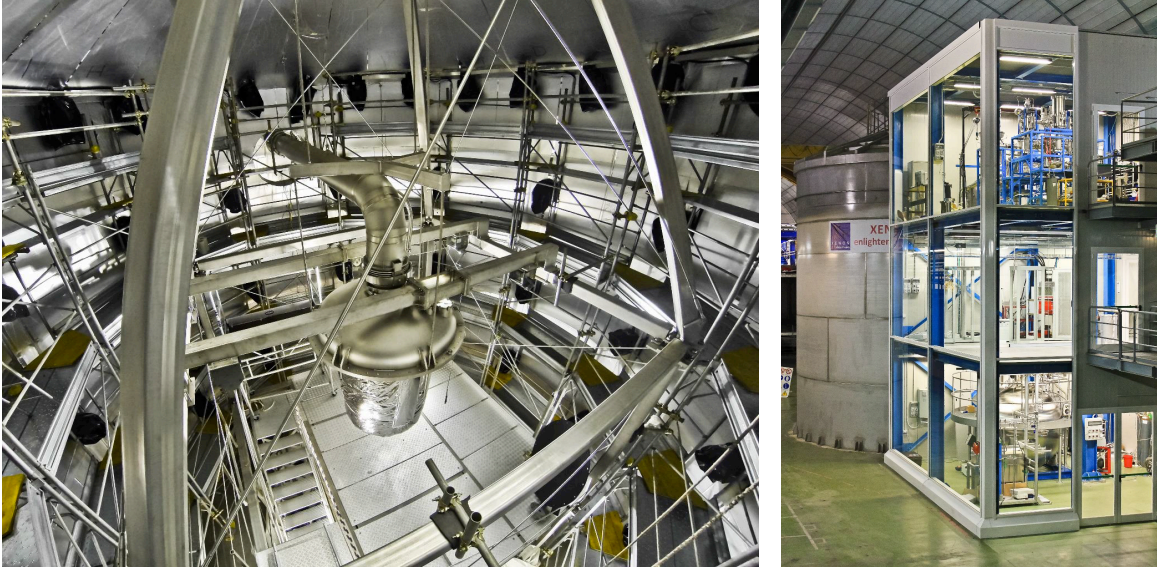
Figure 5: Left: The cryostat of XENON1T with its umbilical pipe, installed on the support structure; the outer thermal insulation vessel is not mounted. The Muon Veto PMTs are also visible, attached to the Water Tank, together with the reflective foil. Right: The service building; on the ground floor the ReStoX and Distillation systems, at floor 1 the DAQ room and at floor 2 the Purification and Cryogenic systems.
