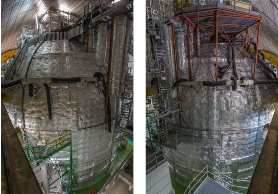
Figure 2: Borexino water tank covered with two layers of 10 cm-thick mineral wool.
