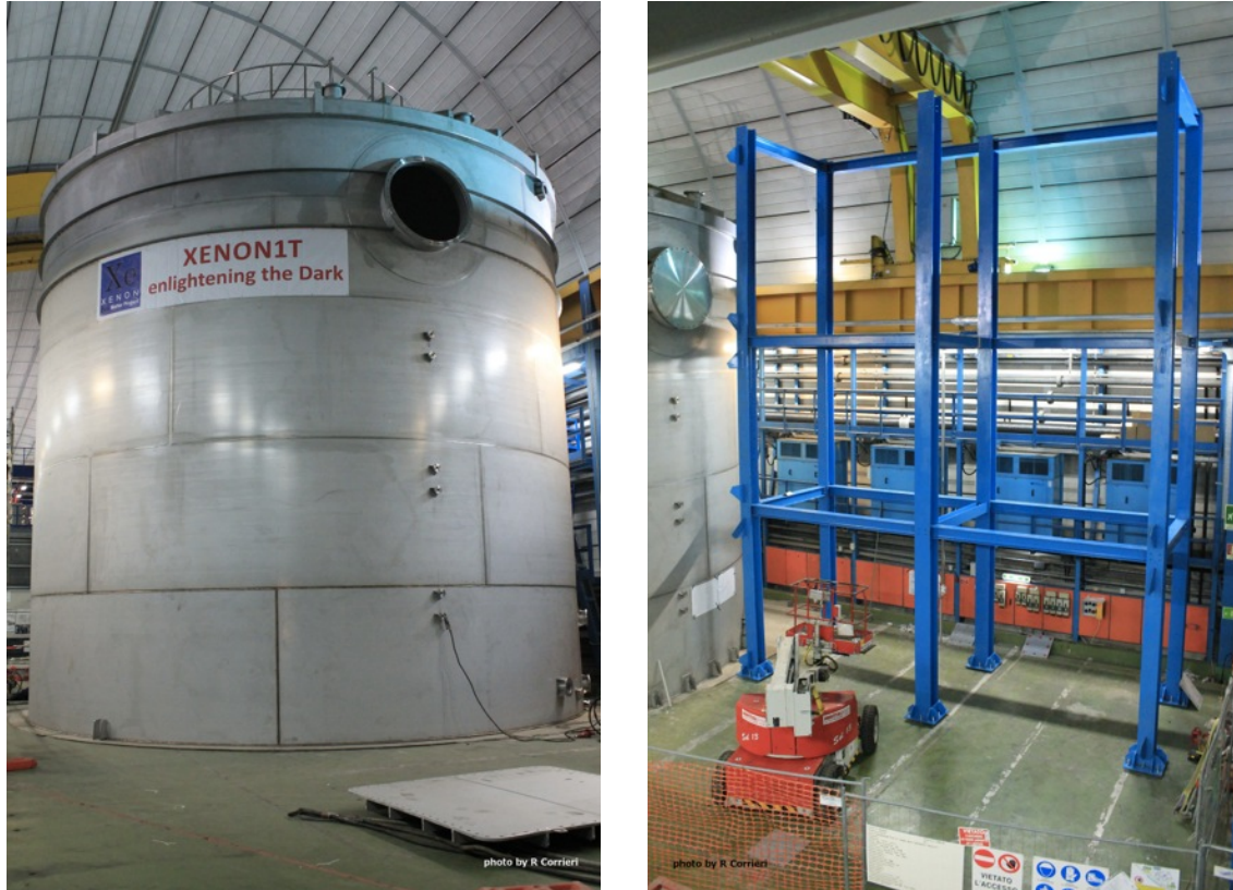
Figure 8: (left) Completed water tank. (right) Raising of the service building.
