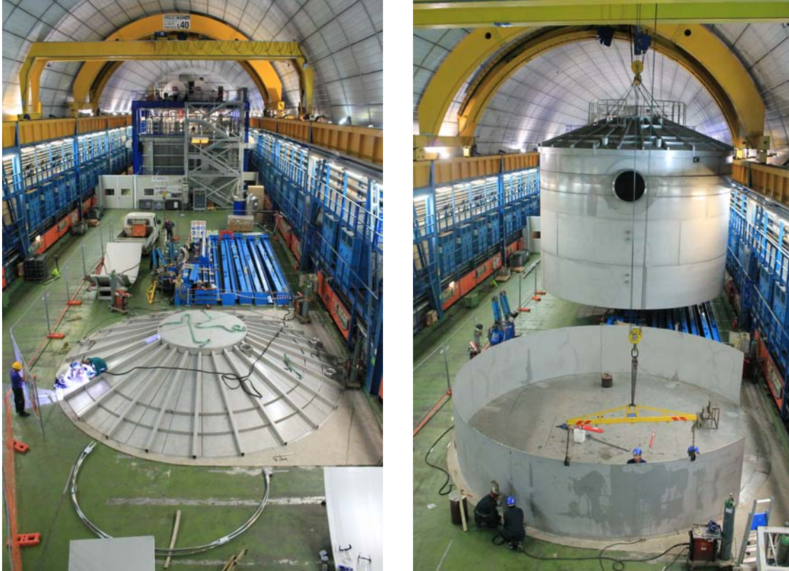
Figure 7: Construction of the water tank in the fall of 2013.
