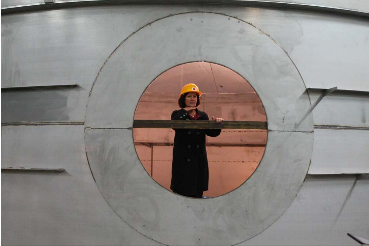
Figure 9: Inspection of the water tank during construction.
