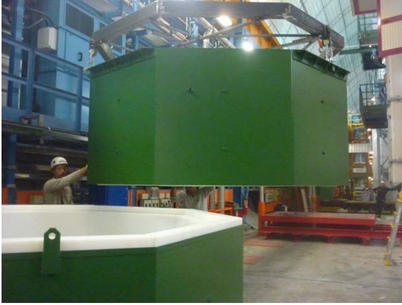
Figure 2: Delivery of the external shield in Hall A.
