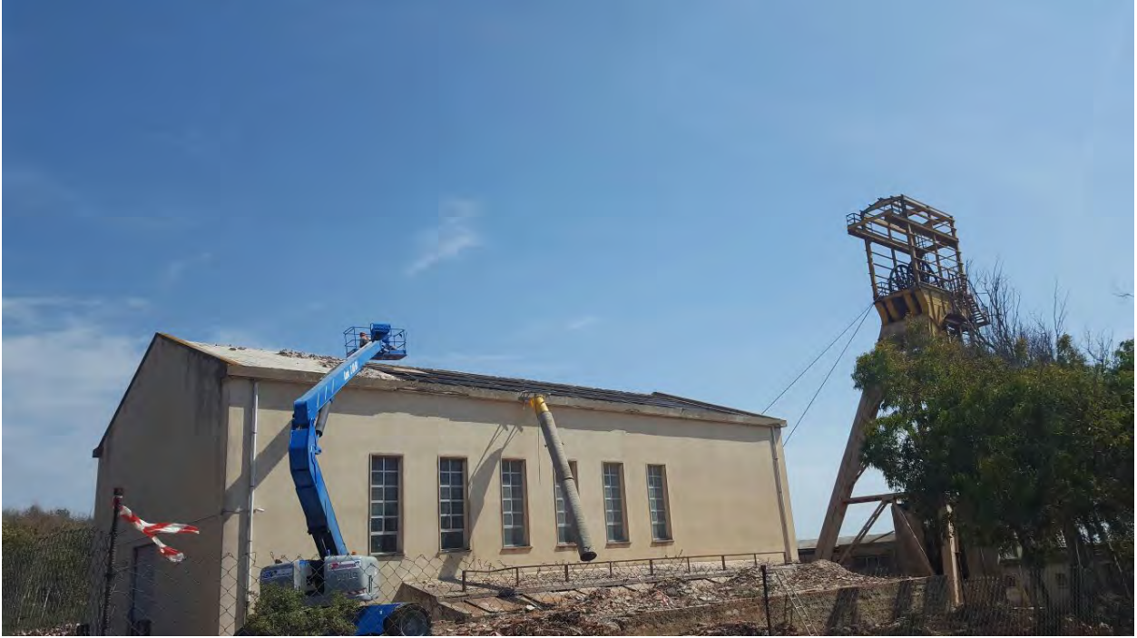
FIG. 11. Aria: refurbishment of the roof covering the Seruci winze building, Summer 2016.
