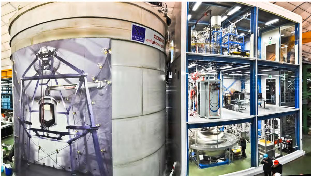
Figure 1: The XENON experiment underground in Hall B of the Gran Sasso lab. On the left the water tank is visible with an attached rendering of the inside, including the heart of the detector at its center. On the right the three-story service building is visible.
