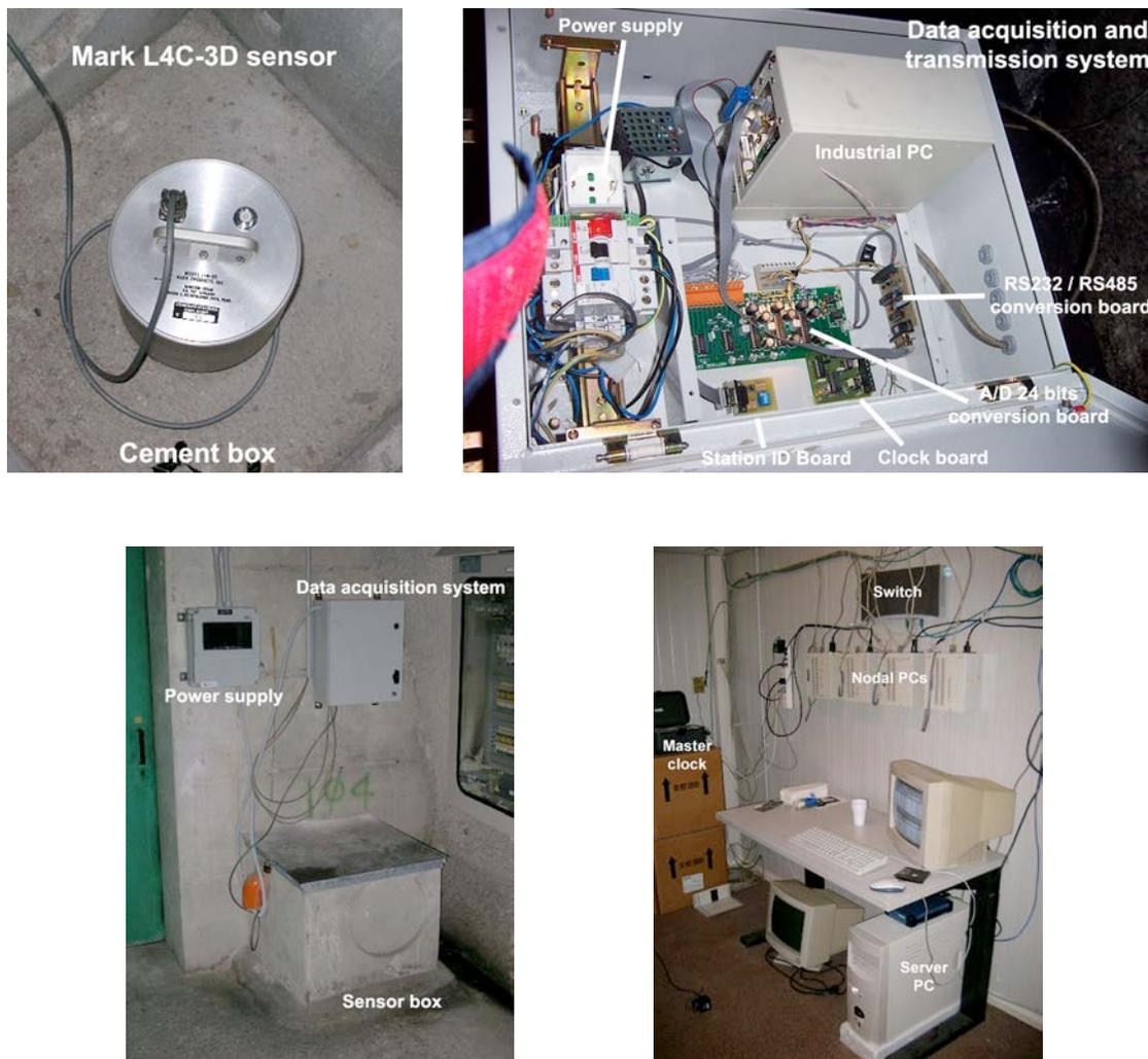
Figure 3: Underground Seismic Array components and control room.
