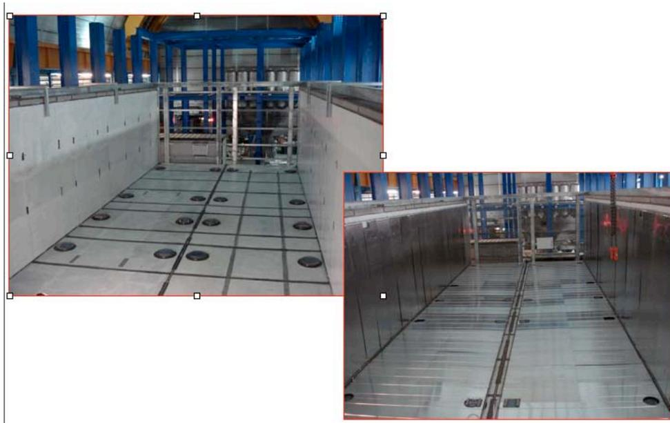
Figure 1: *Picture of insulation panels [Left] and Cold Screens [Right] during the installation inside the mechanical sustaining structure.*
