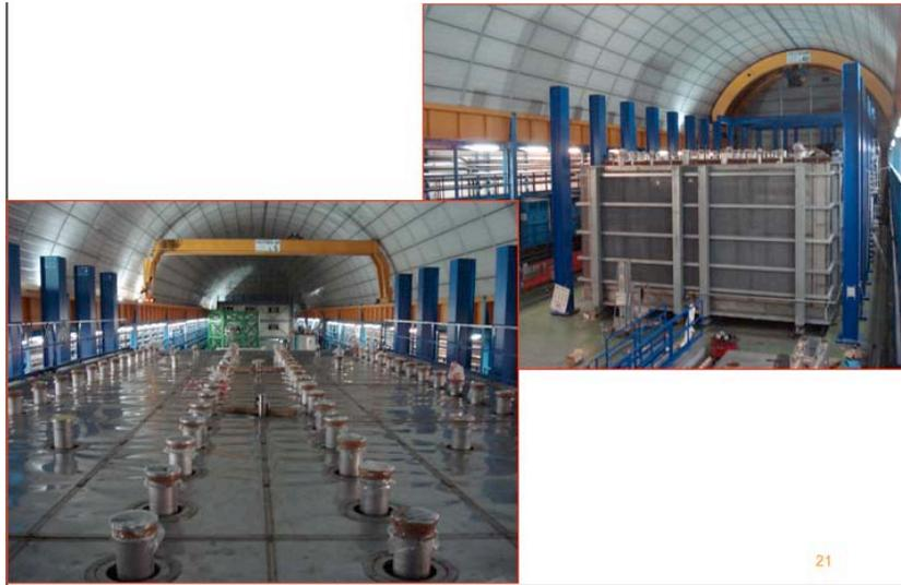
Figure 11: *Top side of the T600 after positioning of the insulation panels..*
