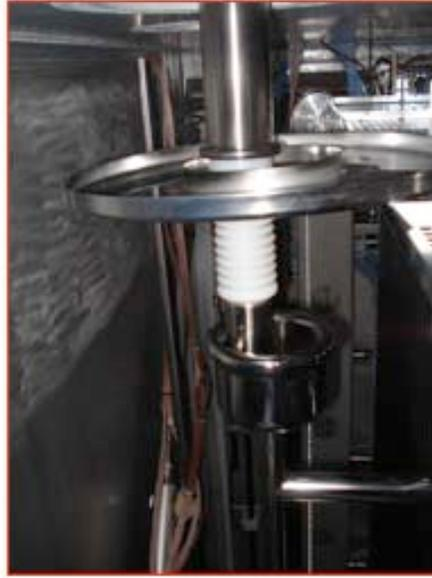
Figure 7: *Picture of the HV feed-through during installation.*
